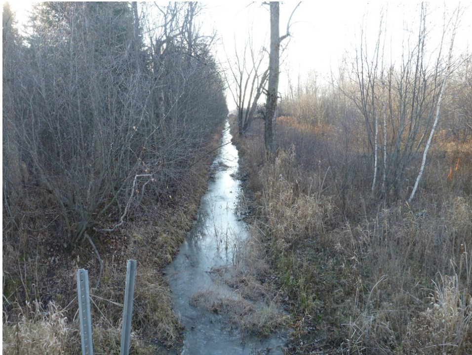
Image 5: Man-made drainage and culvert flowing through the study area, looking west.
