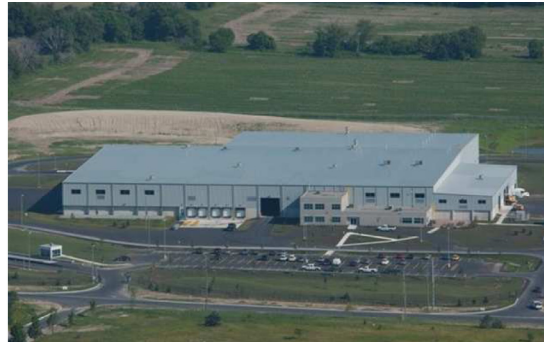
② Material Recovery Facility
