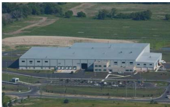
Material Recovery Facility / Centre de tri
